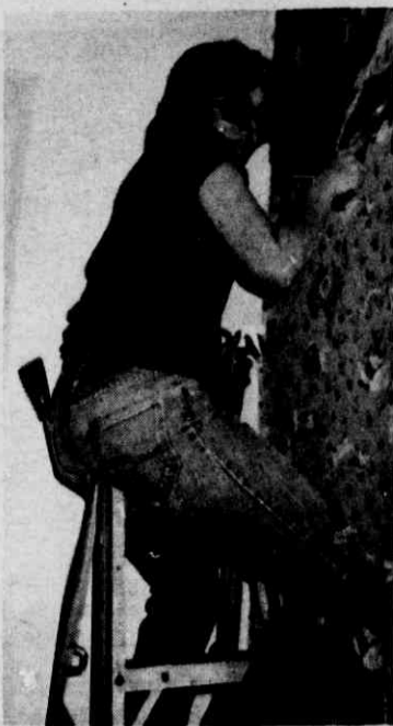
Toby Silber scraping walls at Arosa House.
