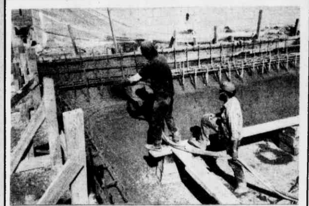
Blowing cement to make walls of indoor pool.
