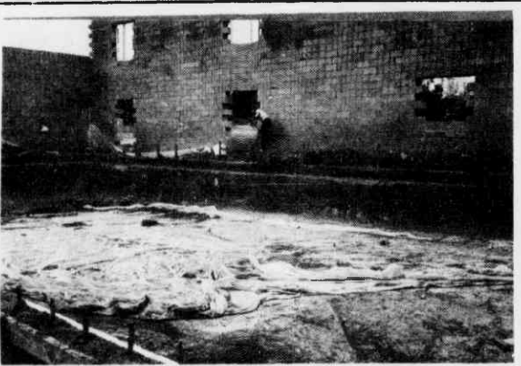
Indoor pool complete with sides now waiting to be tiled.
