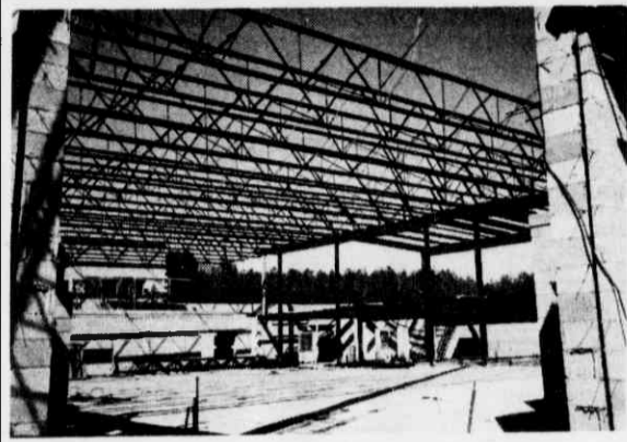
The first long braces in place over the gym.
