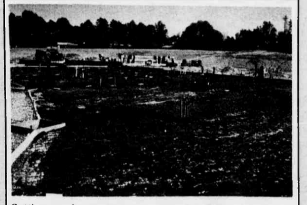
Getting ready to pour concrete for Education Center classrooms.
