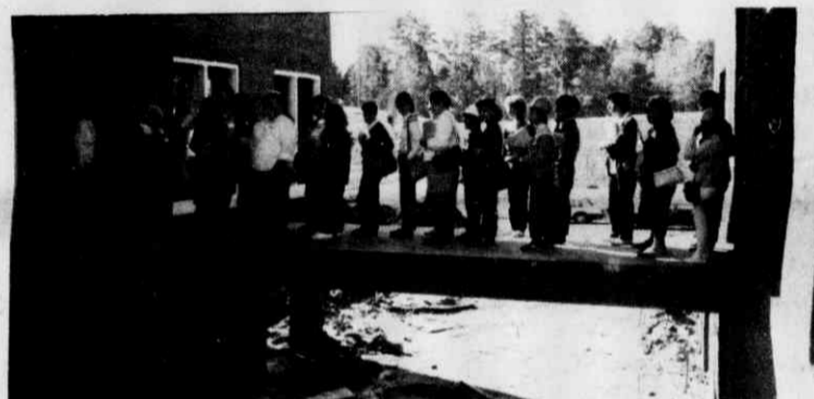
Crossing the bridge connecting the two buildings.
