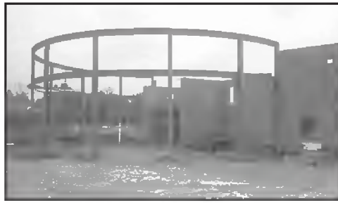
Construction progresses at the Hebrew Cemetery.
