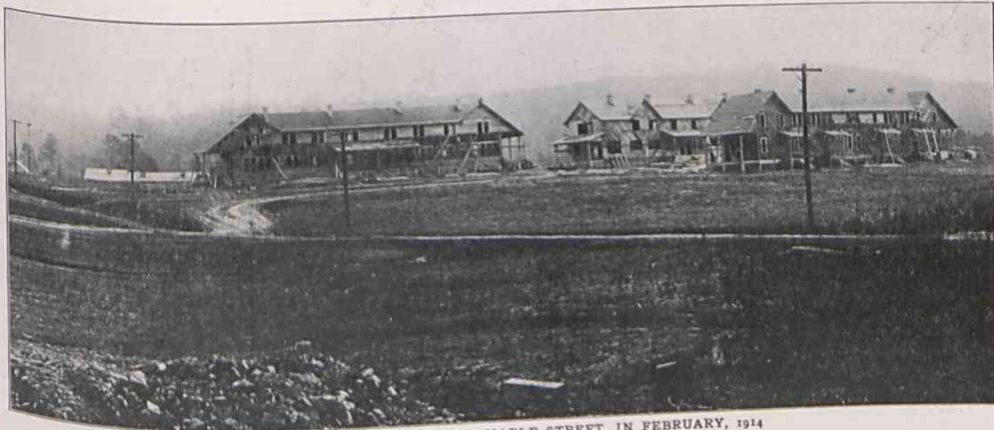
CORNER OF FALLS ROAD AND MAPLE STREET, IN FEBRUARY, 1914
