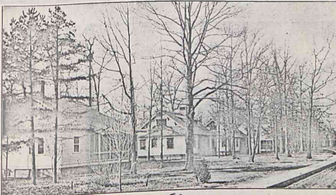
A RESIDENTIAL STREET SCENE
