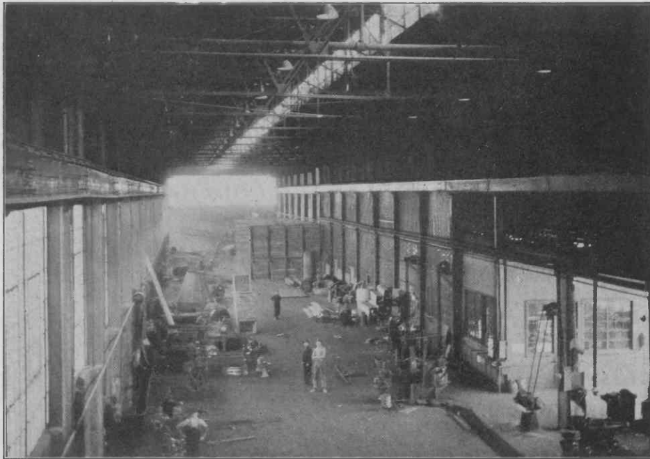
INTERIOR MACHINE SHOP— LOOKING EAST
