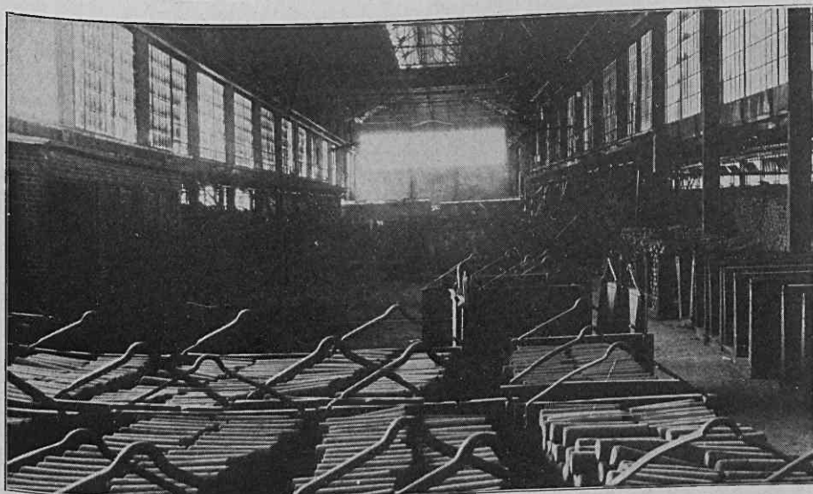
INTERIOR BUILDING 30—CARBON RODDING DEPARTMENT
