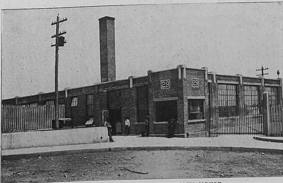
BUILDING NO. 29—NORTH BADIN WASH HOUSE
