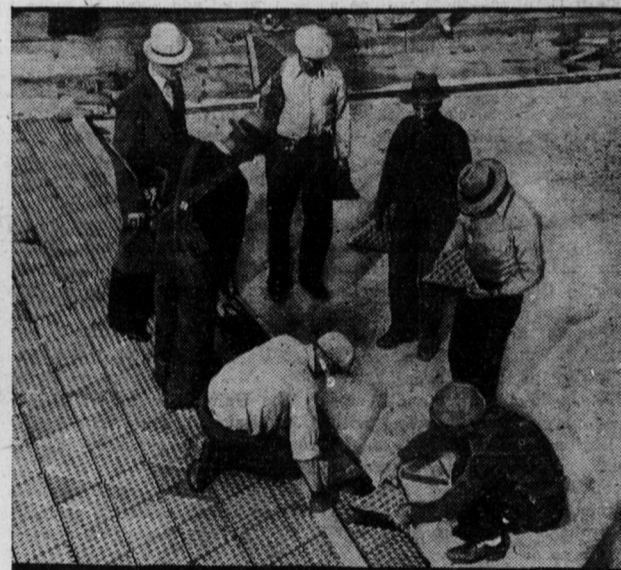
Cast iron paving made its debut in the United States when a thirty-foot strip was laid at the University of Minnesota in Minneapolis for a test to determine its possibilities on a national scale.
