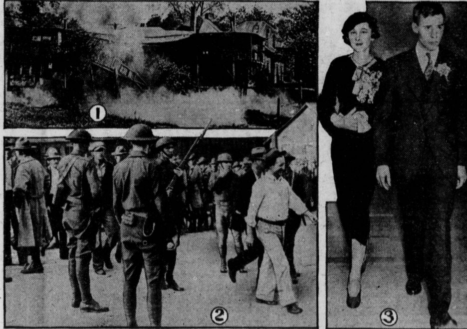
1—Wrecking buildings in Atlanta, Ga., as the government's slum elimination program there was started. 2—Georgia National Guardsmen clearing pickets from stove foundries at Rome to permit reopening of the plants and shipment of goods. 3—Charles Carey Rumsey, Jr., grandson of the late E. H. Harriman, Harvard graduate and polo player, and his bride, who was Mary Maloney daughter of a laundress of East Norwich, Long Island.
