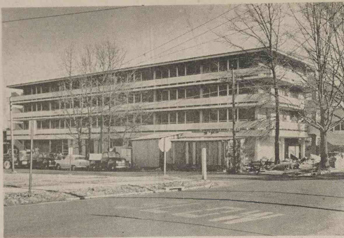
NEW DORM — Now being completed at Deans and Gold Streets, will house 144 men students at Atlantic Christian College. Completion is expected early in the Spring semester. (Collegiate photo by Dee Winstead)
