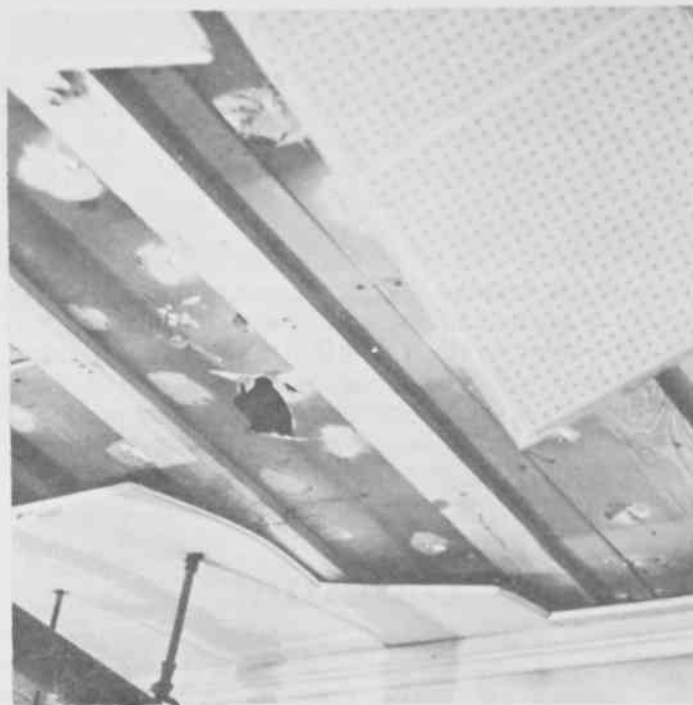
Dressing room ceiling
