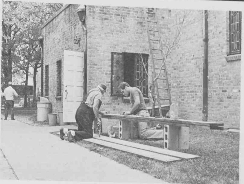
Howard Chapel gets interior face lift.
