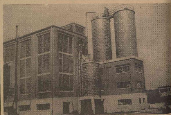
Shown above is the Boiler House and the two large coal silos. The photo in the center is a view of the mezzanine floor under the coal silos, showing the coal scales and screw conveyors. At bottom is a view of the water softeners through which all fresh water makeup must pass.
