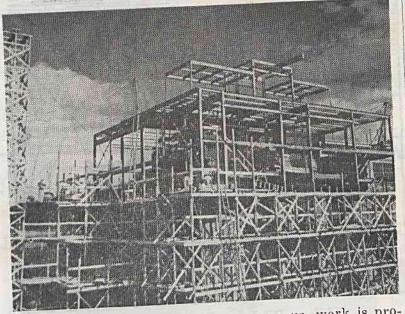
As winter continues to creep up on us, work is progressing rapidly on the extension to the boiler room. This new addition will add materially to the capacity of the boiler room. The extension is 65 feet wide and 70 feet long.
