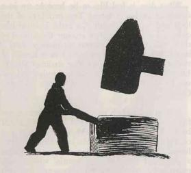
Shown at top right on the facing page is a picture of the Big Hammer. Below is a drawing of the hammer, showing how it was used to beat the strips of manganese. The spikes in the waterwheel caught the end of the handle, pushed it down and released it as the wheel continued to turn.
