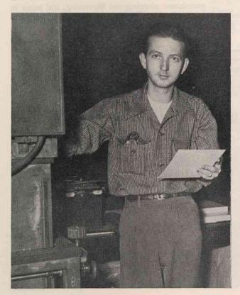
Ted Mull, photo-lithographer. Ted handles the entire process of plate making from the initial step of photography to the point of press operation.
