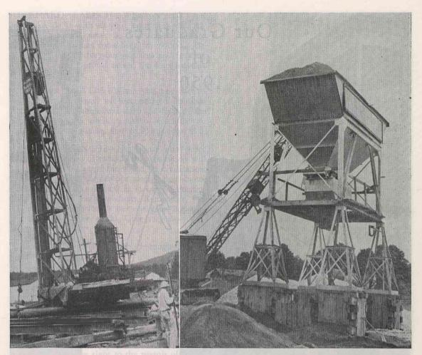
Above, left: Shown in the picture is the MacArthur Pile Driving Rig which is a patented cast-in-place concrete foundation pile. A steel mandrel of the desired piling diameter is driven into the ground by steam hammer until proper loading conditions are secured. The mandrel is then withdrawn and freshly mixed concrete poured into the hole made by the mandrel.
