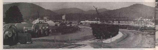
Above: View of one of the railroad spurs. Tanks in left foreground are absorbers for coating solvent recovery.
