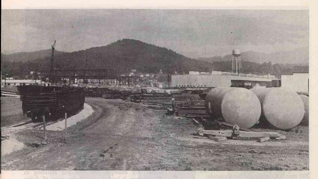
Above: Another view of the tank storage and steel sorting area. Tanks in right foreground are carbon bisulphide storage tanks.
