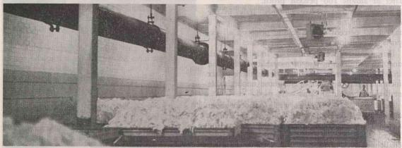
ABOVE: Process steam and steam for prime movers is piped directly from the existing boiler plant to the cellophane operation. Note the 20" welded steel overhead steam line on left hand side of the photograph as it passes through the pulp storage room.
