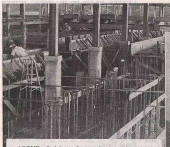
ABOVE: Bedplates for casting machines have already been partially installed. This photograph shows the intricate re-inforced interior foundations for casting machines No. 6 and No. 7.
