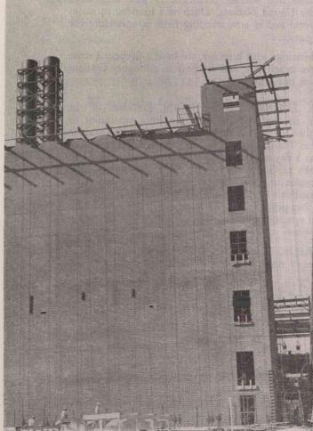
ABOVE: With Solvent Storage tank foundations shown in the foreground, this eastward view pictures Du-Pont forces pouring the upper floors of the Solvent Recovery Building. Note the large bucket lifted by the crane to supply concrete for this operation.
