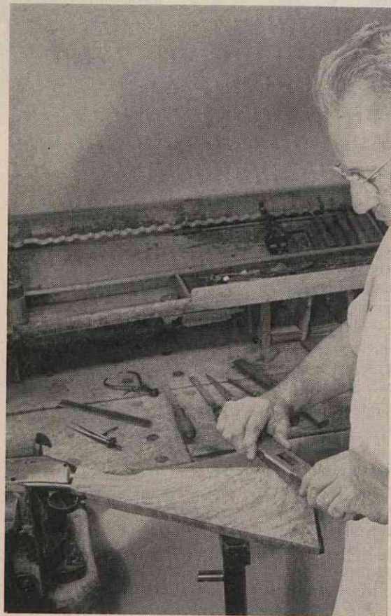
Above: The steps in the making of the pistol grip stock and forearm for the Model 21. Selected, top grade American Walnut is used.
