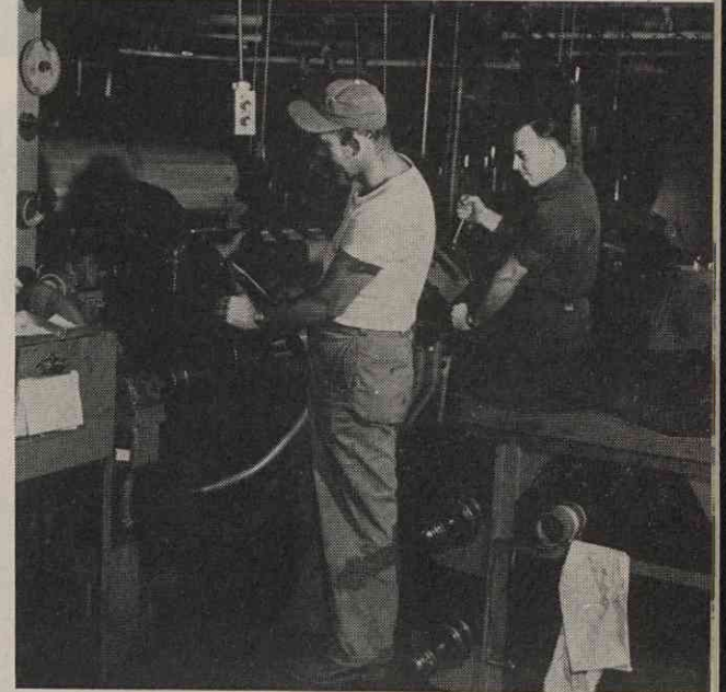
↑ Clyde Whittington and Leroy Mills are repairing the grab-hoist which is above slitting machine.
