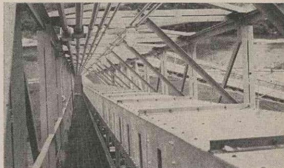
At left is shown the coal conveyor in the tunnel as it carries the crushed coal from the crusher to the Boiler House. Above is the conveyor and walkway from the Transfer House to the top of the Boiler House. This photo was taken from the Boiler House roof looking downward. The conveyors and walkways rise at an angle of about 17 degrees with the ground.
