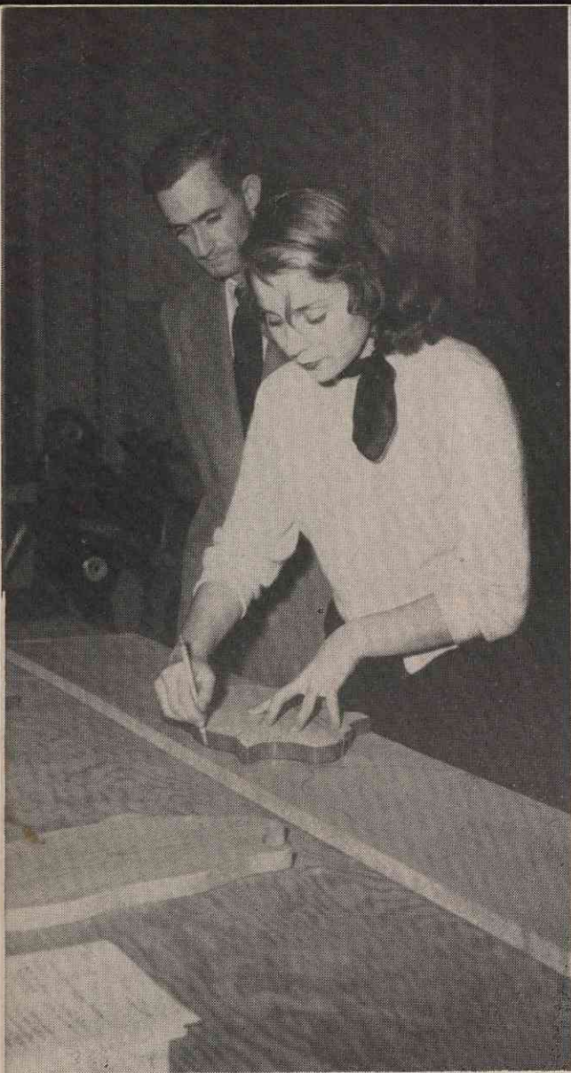
Left: Earl York checks on Nelle Cherry's progress as she outlines a design of the Blue Ribbon Piggy (Hammus Carolinus variety) Board on a hardwood board. The boards are then given to the jig saw operator who seperates the designs and saws the boards to conform to the outline. Above: William Walters uses the jig saw to cut out the chopping boards as Jim Willis looks on. Achievers take a turn in every production phase.
