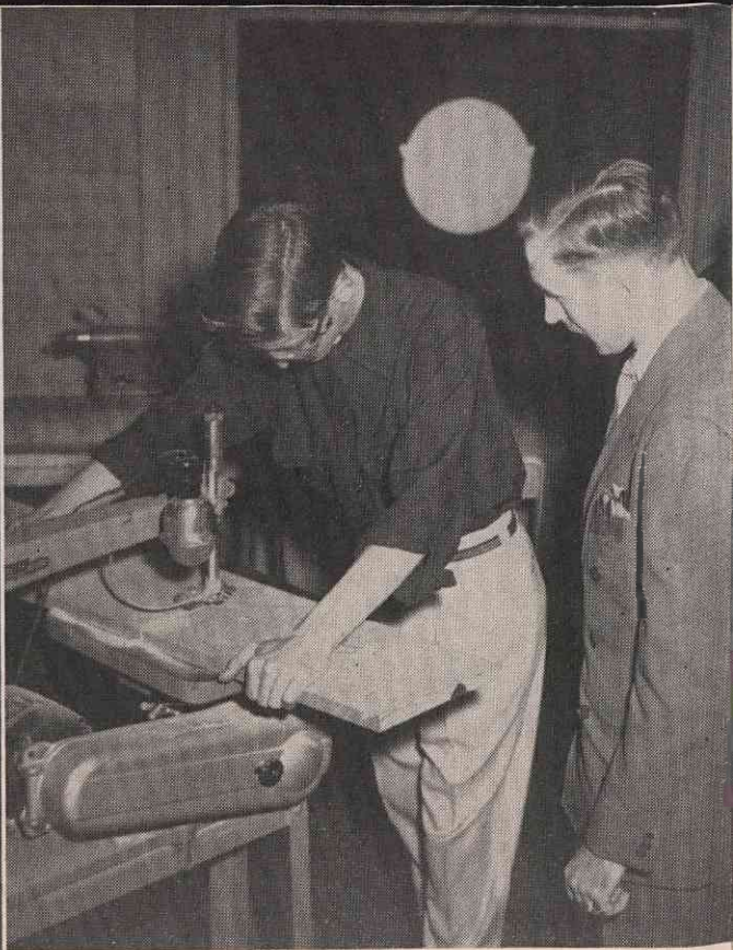
Left: Earl York checks on Nelle Cherry's progress as she outlines a design of the Blue Ribbon Piggy (Hammus Carolinus variety) Board on a hardwood board. The boards are then given to the jig saw operator who seperates the designs and saws the boards to conform to the outline. Above: William Walters uses the jig saw to cut out the chopping boards as Jim Willis looks on. Achievers take a turn in every production phase.
