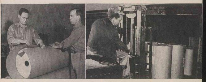
Horace Lancaster and Ernest Lyday carefully wrap the slit rolls in corrugated cardboard to prevent possible damage during shipment to the Paas Co.
