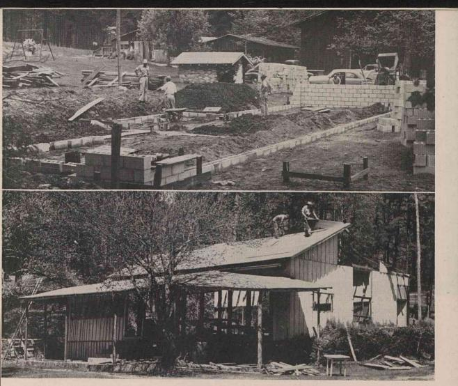
Top: A photo of the new canteen-bathhouse three days after the start of construction. Walls of the structure are of cement block and floors of all three sections will be of poured concrete. In
