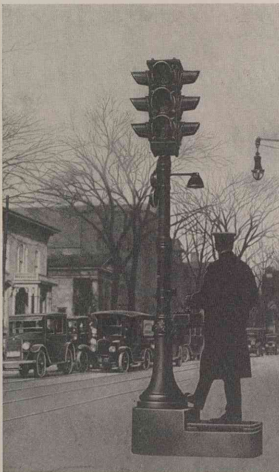
In the passing scene we saw the world's first installation of a 4-way 3-section traffic signal in 1922, Syracuse, New York.
