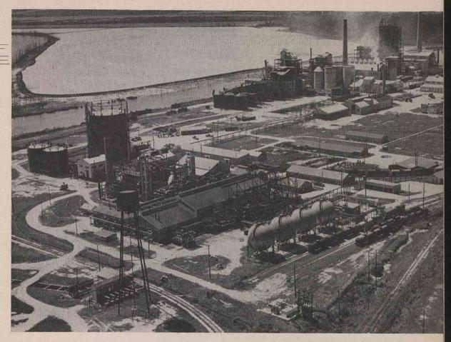
dissolve the salt. The brine is then pumped through a pipeline to the plant where it is purified, ammoniated and mixed with the carbon dioxide in large towers.
