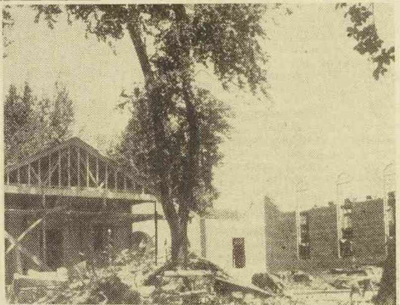
Methodist Church Rapidly Progressing
