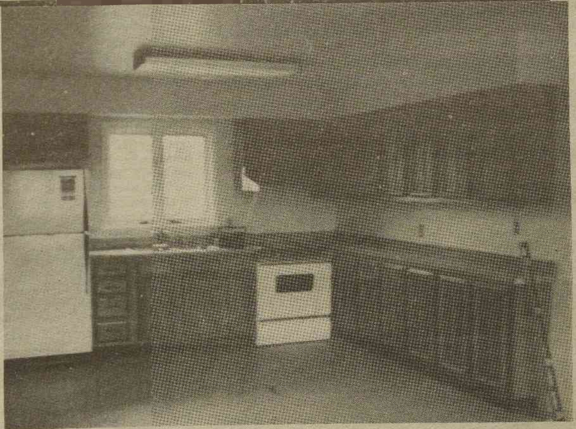
In the final stages of completion, the new apartment complex consists of two spacious kitchens, each featuring a refrigerator, stove, and plenty of cabinet space. For a view point on the additional student housing, see page 2.
