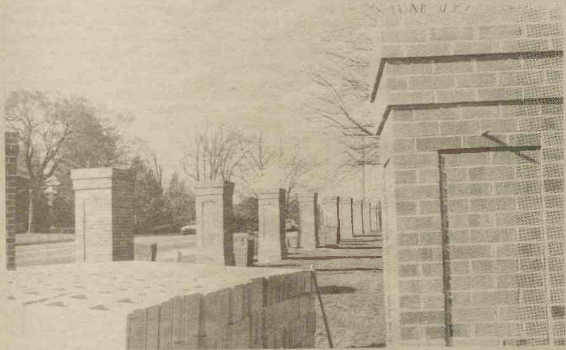
Above is the "Brevard Wall" currently nearing completion.
