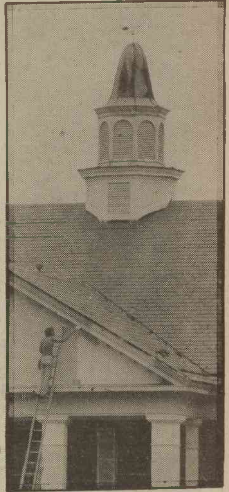
More changes around campus — repainting the buildings
