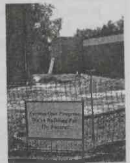
Construction seen from the academic quad.
