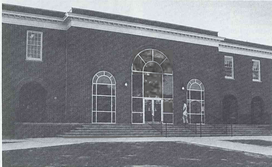
The new entrance of Randall Library faces the Social and Behavioral Science building. The library gained 23,500 square feet, has seating space for 950 students, and can accommodate 475,000 books.
