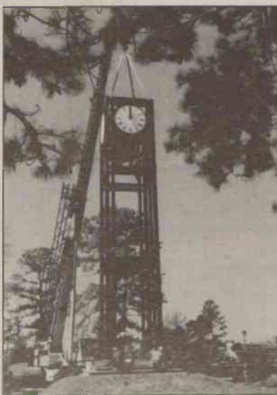
A crane lifts the tower into place atop its foundation May 11.
