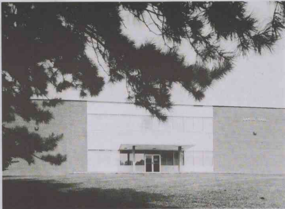
Daniel Hall, named in memory of Professor Jeannette Snead Daniel, is slated for renovation and improvements.
