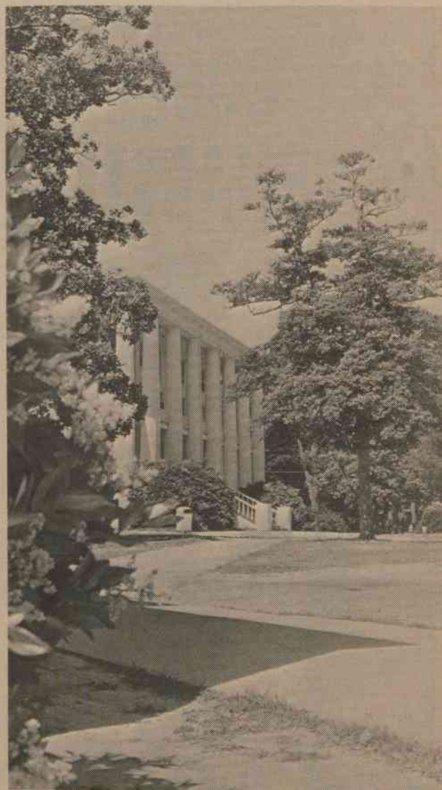
THIS COULD BE a scene from 1851 when the Chowan Baptist Female Institute first opened the doors of the Columns. Instead, it's summer, 1970. McDowell Columns Building is a favorite of visitors to the campus.
