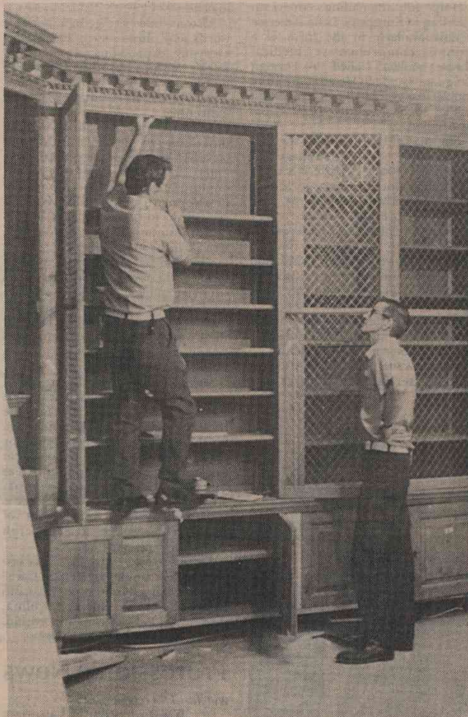
PUTTING IT BACK TOGETHER AGAIN —Piece by piece, the antique white pine paneling and moldings of the Trent Room were brought the quarter mile from the medical center's library to their new home in the almost completed communications center. Carpenters J. T. White, right, and Pedro Seagroves have spent the better part of the past month painstakingly recreating the room, which houses rare books. (Photo by Margaret Howell)
