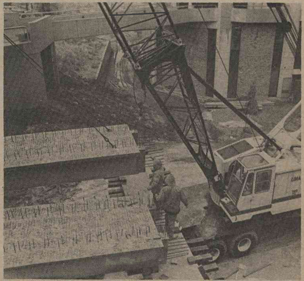
BRIDGE BETWEEN TWO HOSPITALS—A crane and several workmen install a section of the bridge which will carry the personnel rapid transit (PRT) across the deep ravine between the Bell and Mudd Buildings as it runs between the present hospital and Duke Hospital North. Even though the PRT guideway has not been completed, its north-south path is now quite evident. Another chapter in the Duke Hospital North story will be presented in the second edition of "Looking North," which will be published with Heartbeat Feb. 22. (Photos by John Becton)
