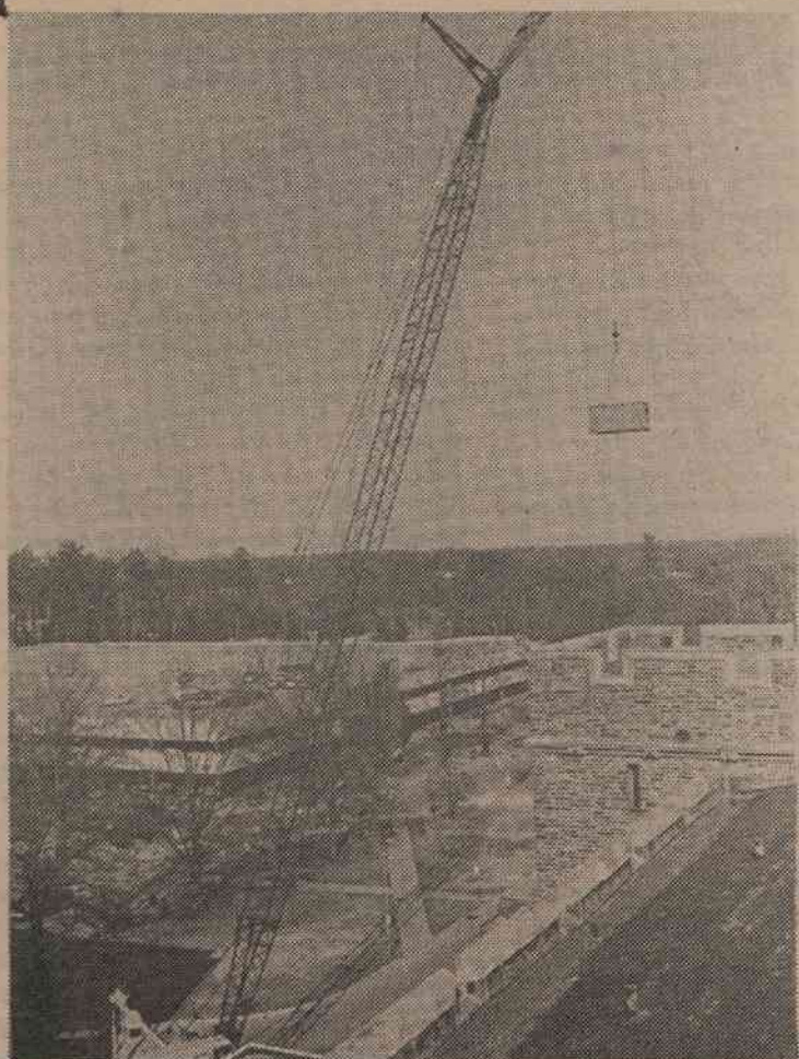
UP, UP, AND OVER!—After a trial run, the air conditioner (see photos on page 1) was attached to the boon with hooks and lifted up over the hospital's front entrance and into the well above the
