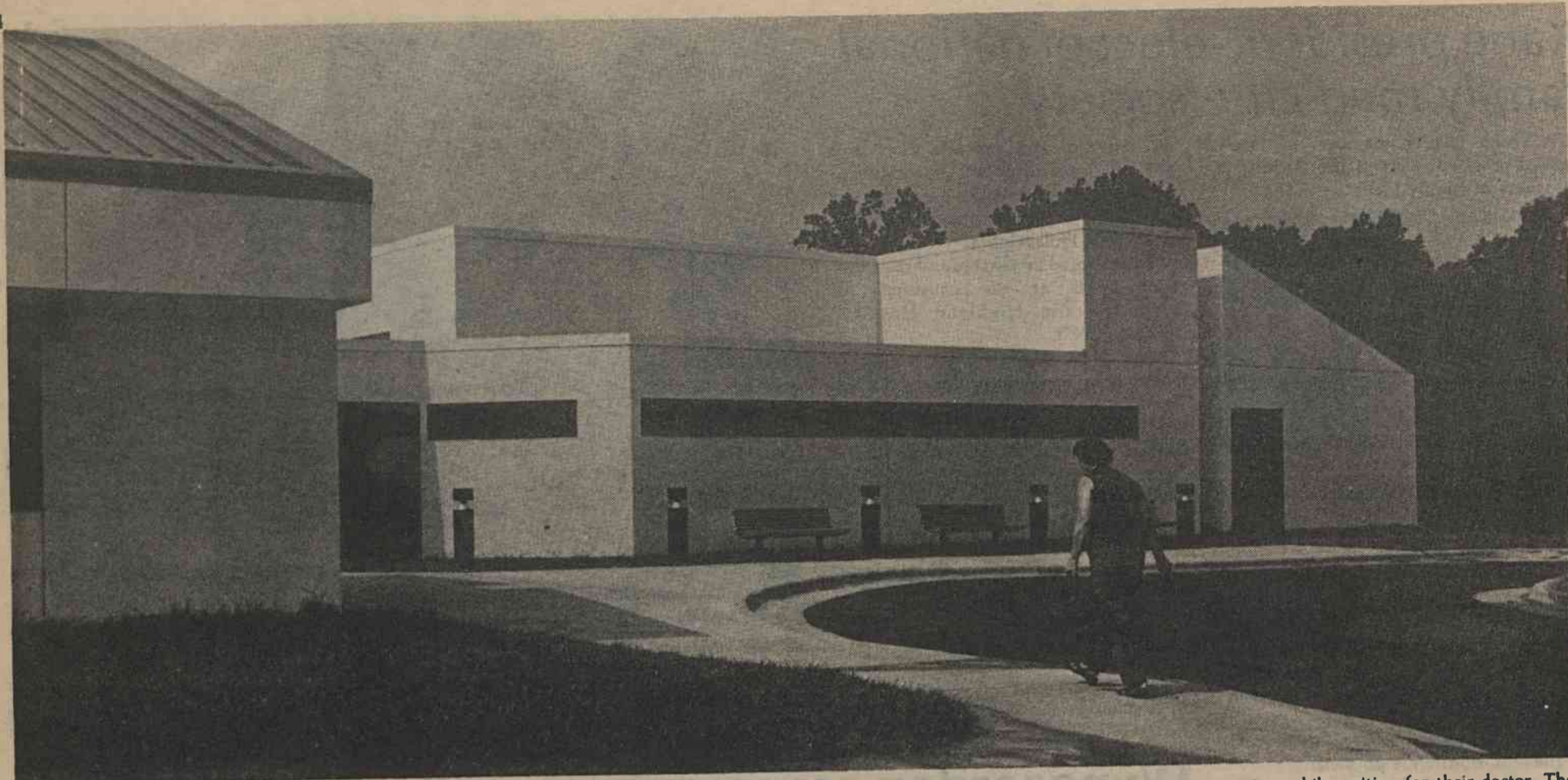
NEW HOME FOR FAMILY MEDICINE — A patient walks up the main entrance of the new family medicine center, located on Crutchfield Street, adjacent to Durham County General Hospital. The new 23,000-square-foot building houses the administrative and clinical portion of the Duke-Watts Family Medicine Program. The formal dedication for the $1.4 million building will be in the
