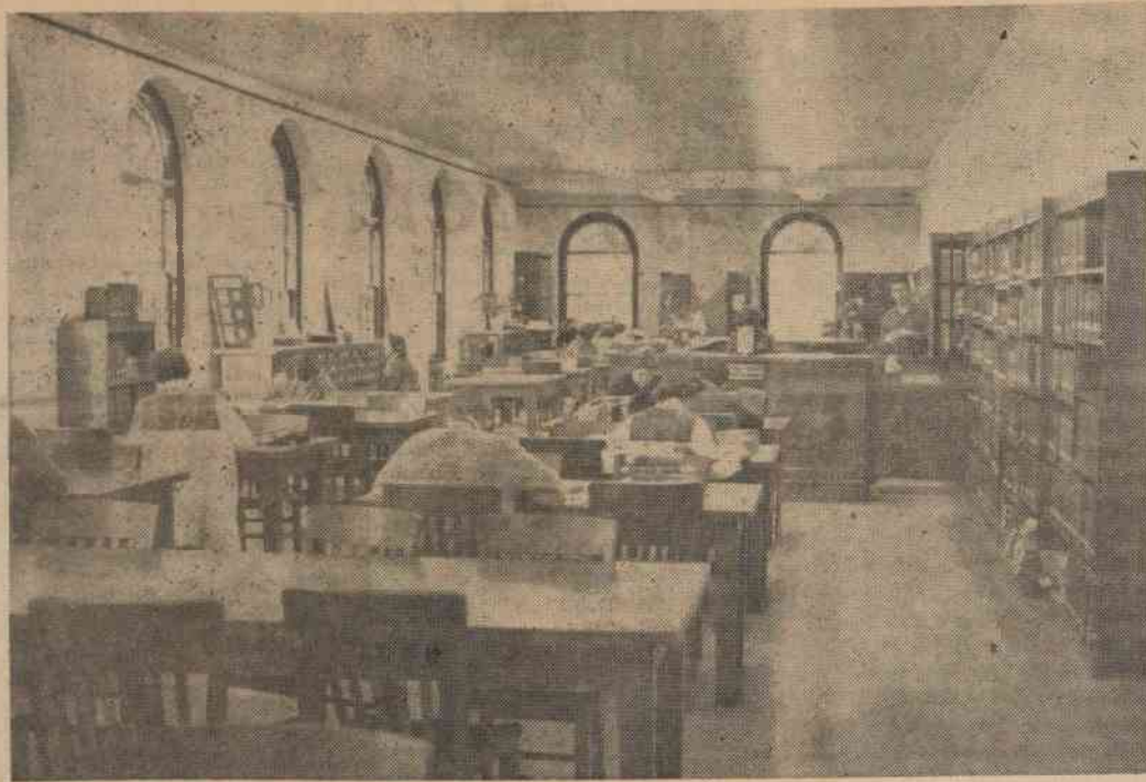
One of the many improvements on the Elon campus this year has been the improved lighting in the college library. The above picture shows the well-lighted reading room of the library since the installation early this year of the new fluorescent lights. Similar lighting fixtures were placed in many of the classrooms on the campus, and plans call for the same improvement in all classrooms as soon as possible.
