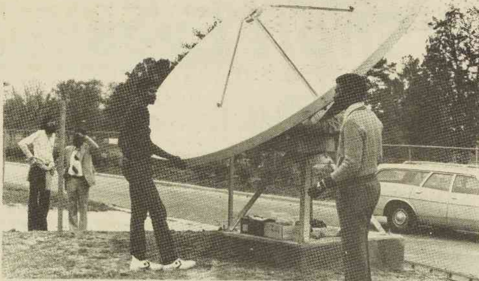
Satellite Receiving Dish being erected next to the Science Complex. This piece of equipment will give WFSS a direct link to National Public Radio via communications satellite.
