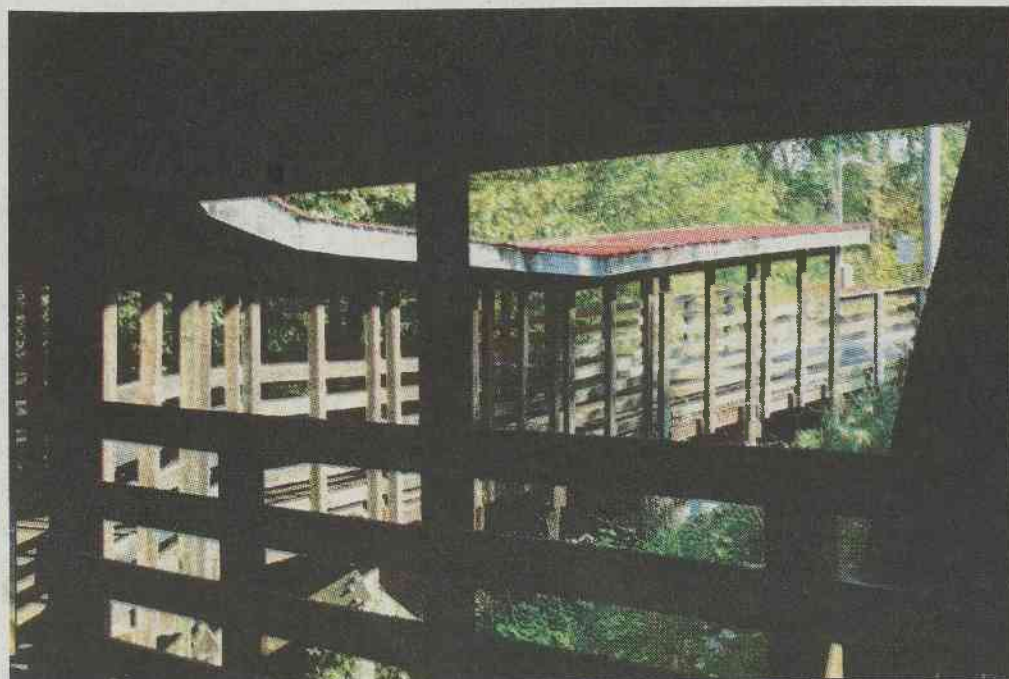
The covered bridge on the Cape Fear River Trail in Fayetteville
