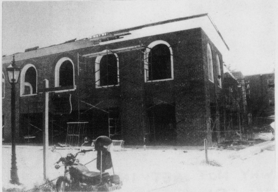
Cafeteria construction continues.
