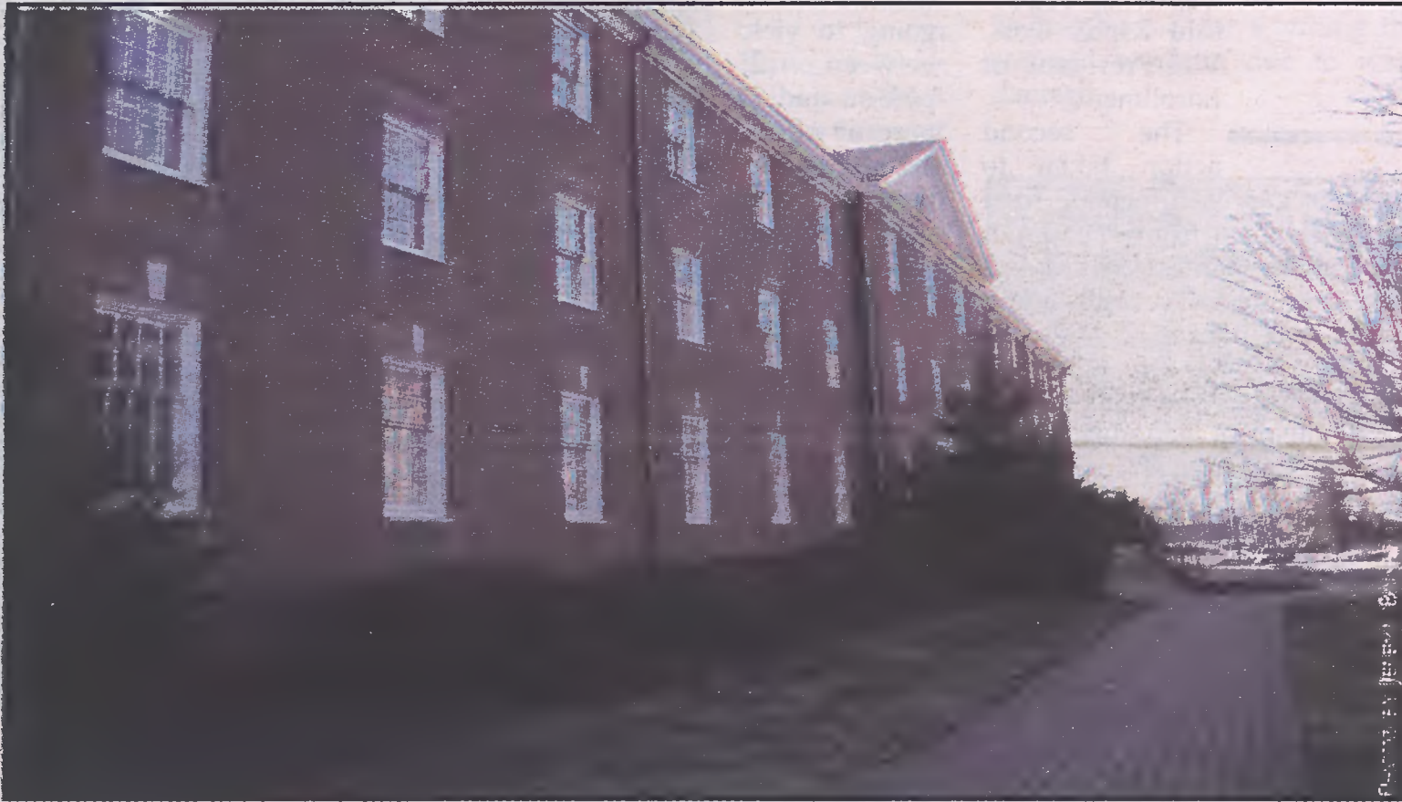
Corroded pipes in Binford break, displacing students.
